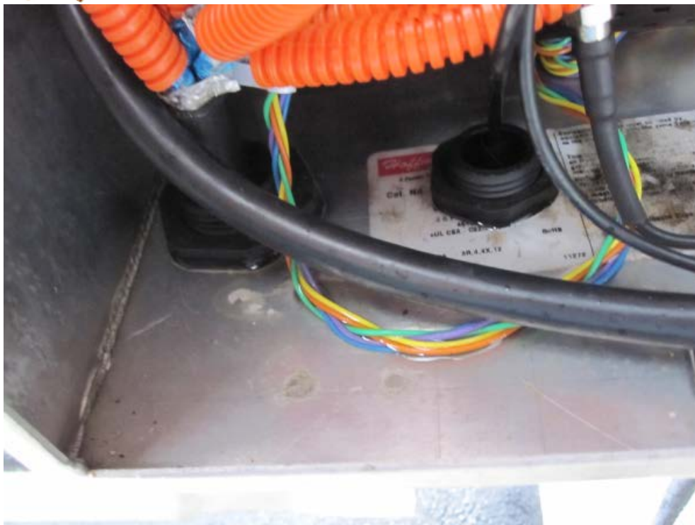
Figure 7 - pooling at bottom of topside enclosure
