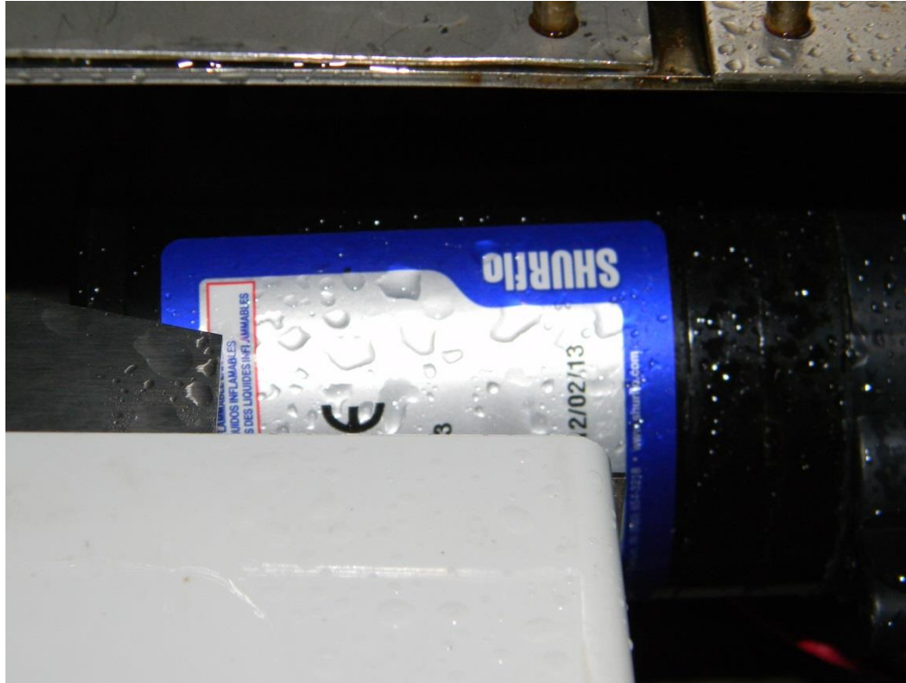
Figure 4: Water spray on pump housing
