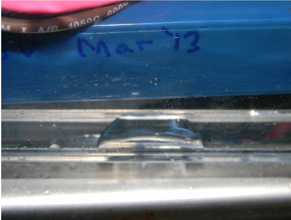
Figure 10: Water inside Pump Control Box
