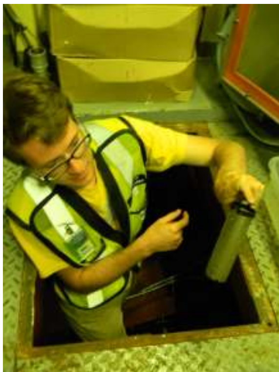
Figure 7: Sea strainer inspection
