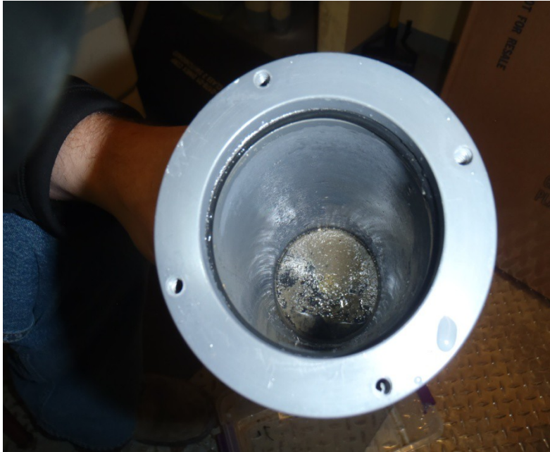
BBFL2 Eco Triplet residue / sediment in housing prior to servicing
