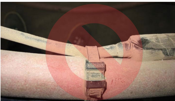
Figure 11. Do not use Zip-Ties Directly on Cables
